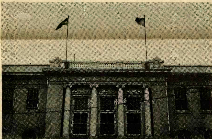
Tierra Amarilla Courthouse
